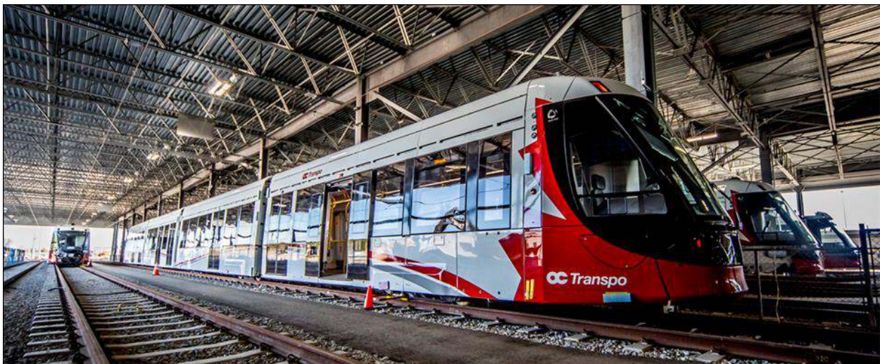
Figure 2: Belfast MSF Expansion: Interior of the New Maintenance Facility
