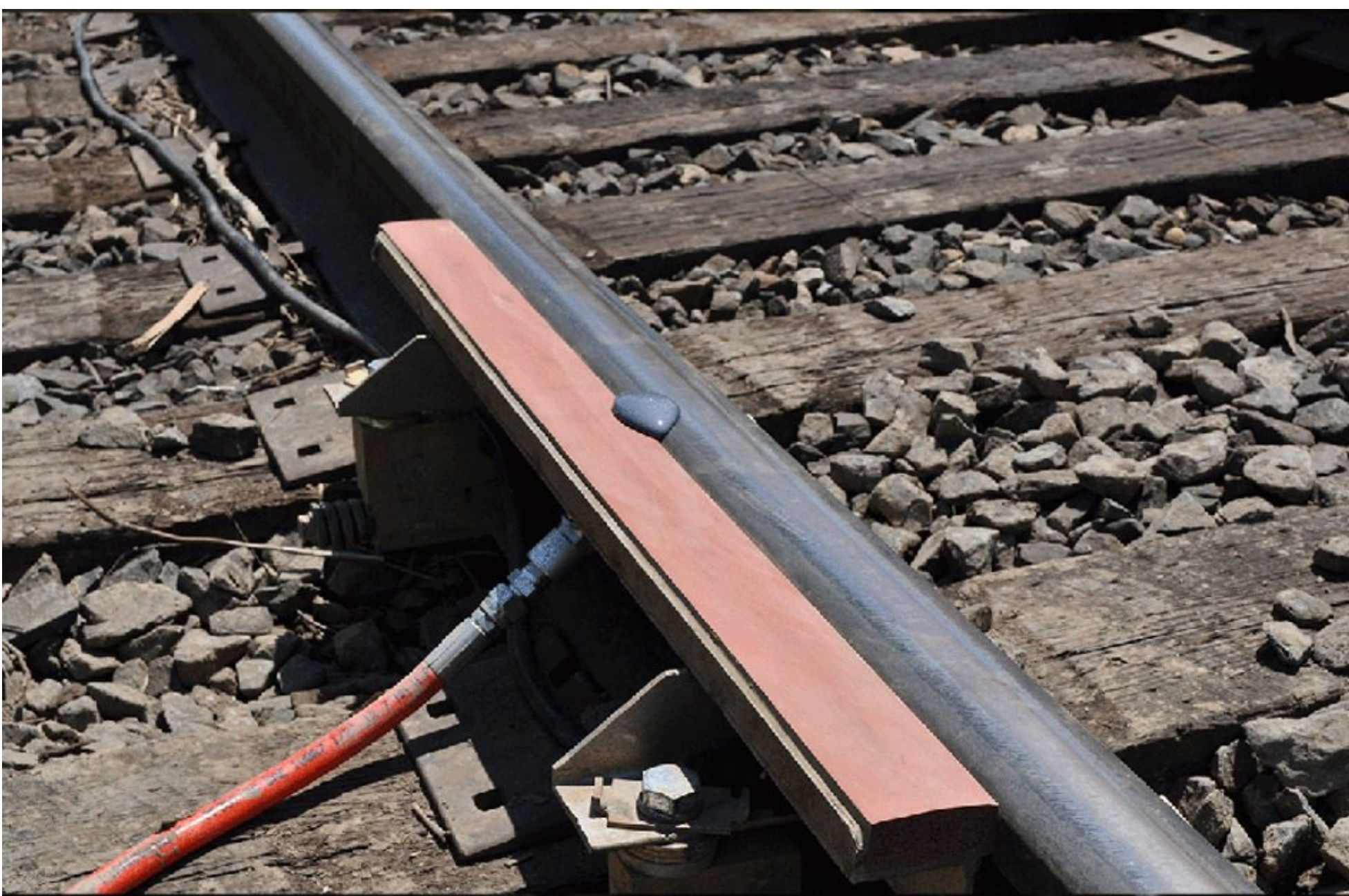
Example – top of rail friction modifier (credit: LBFoster.eu)
